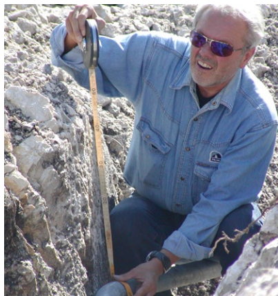
Luciano Lazzaro during slope construction
